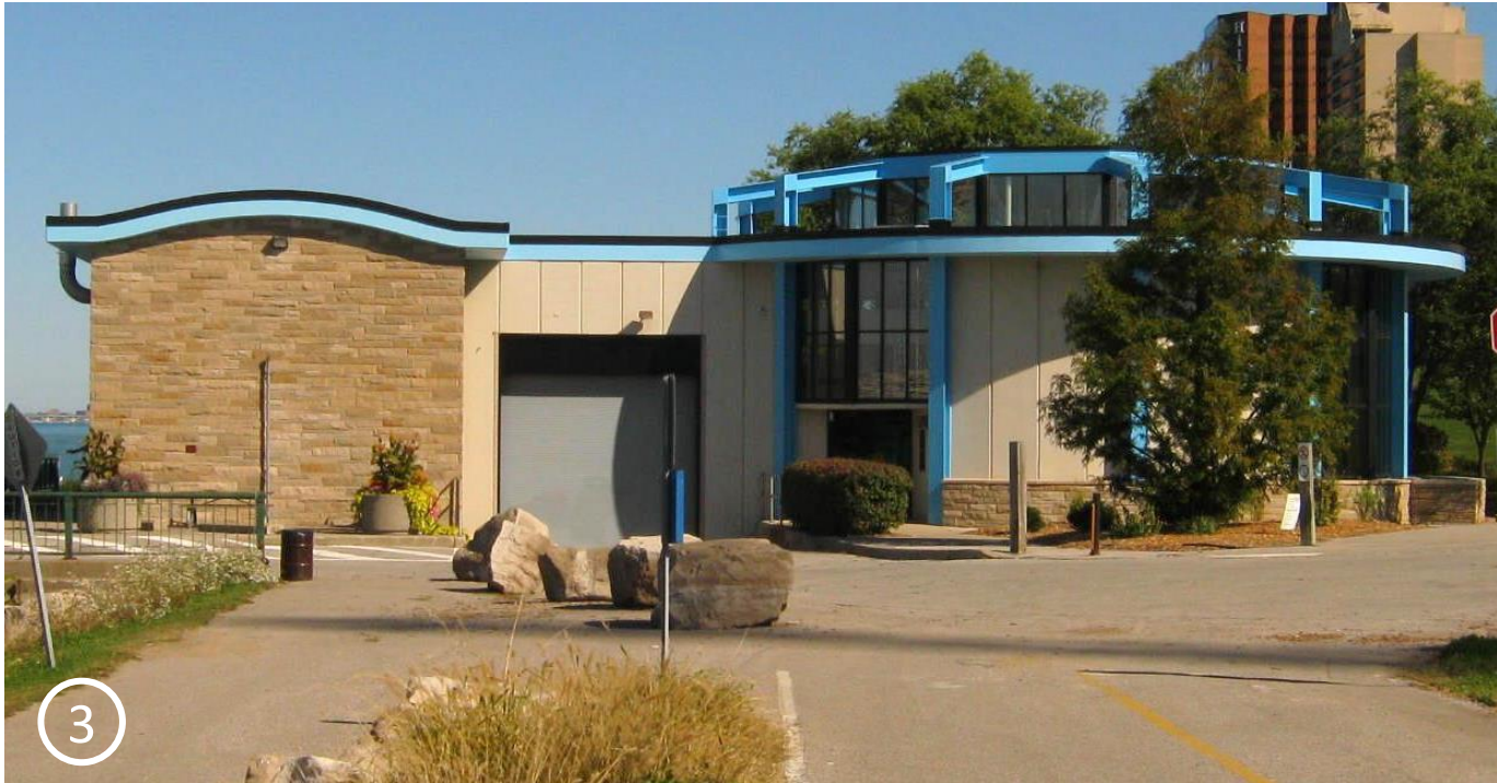
CARON AVENUE PUMP STATION
