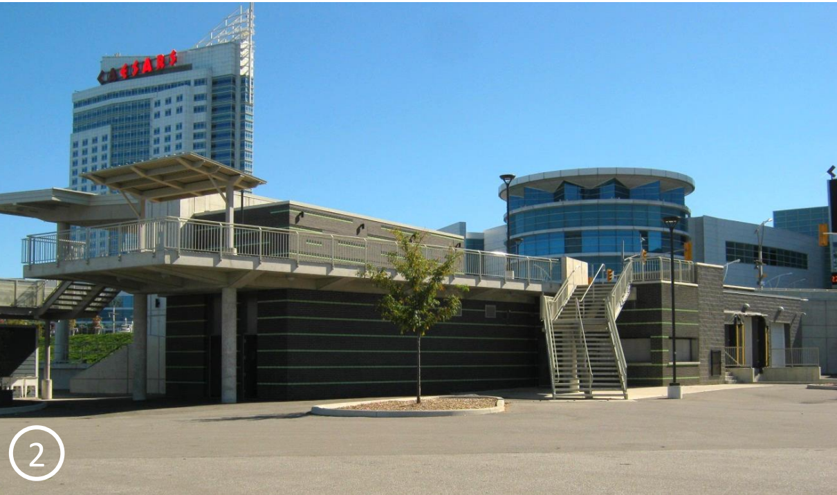
LOOKOUT AND STAIR ACCESS BEHIND COVERED STAGE
