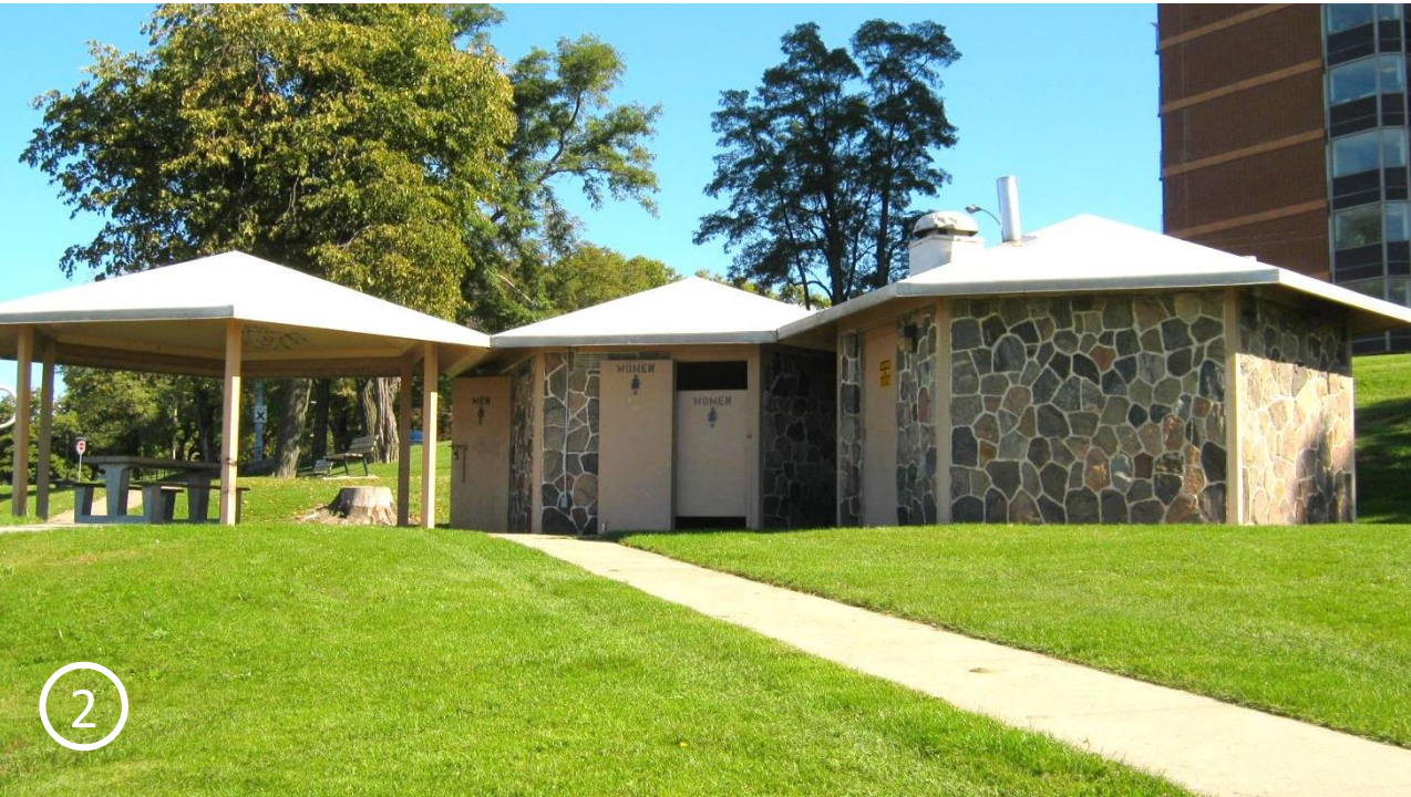
EXISTING WASHROOM BUILDING
