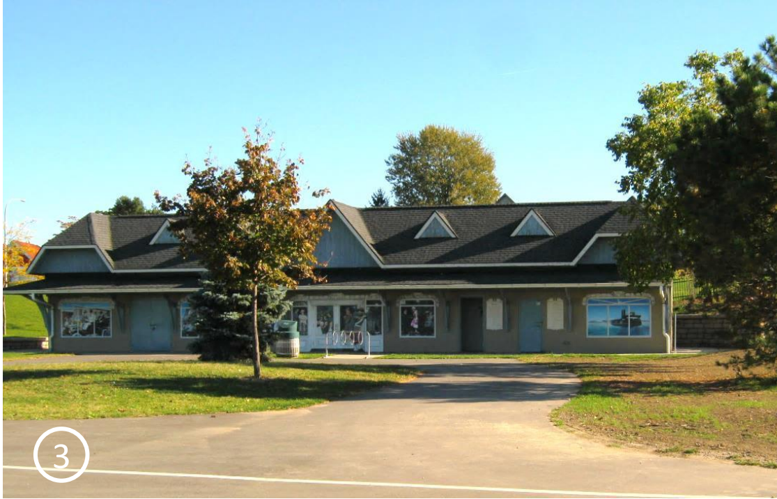
WASHROOM AND MAINTENANCE BUILDING
