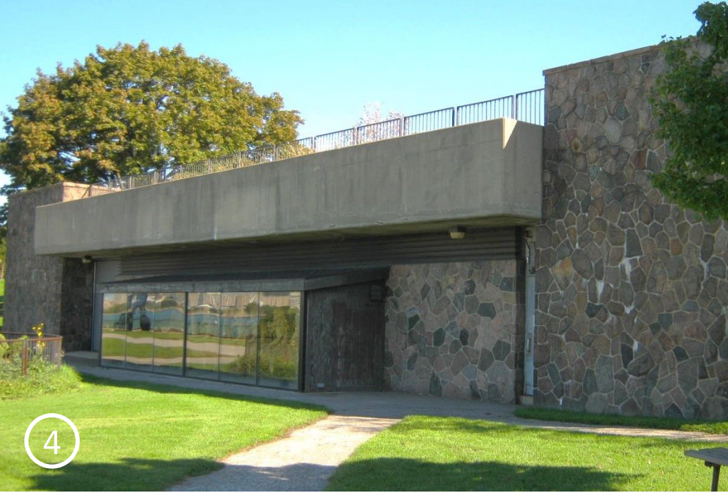
UNIVERSITY PUMP HOUSE
