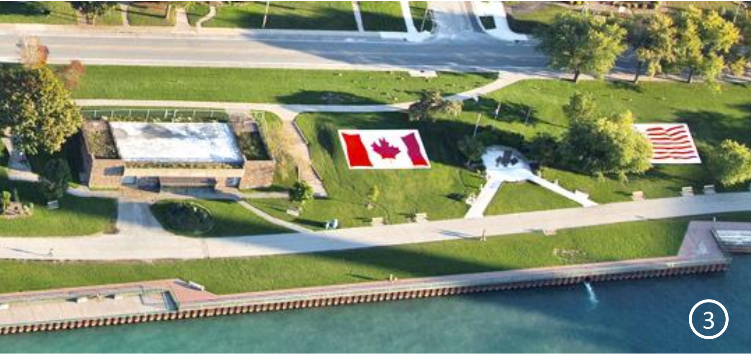
UNIVERSITY PUMP HOUSE & VIETNAM MEMORIAL COURT
