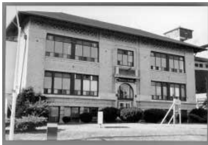
Ford City School, 1917 3177 Riverside Dr. E. (Demolished)
